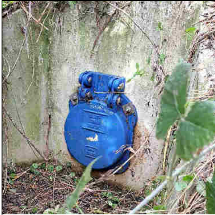
Photograph 15: Backflow Prevention Cover
